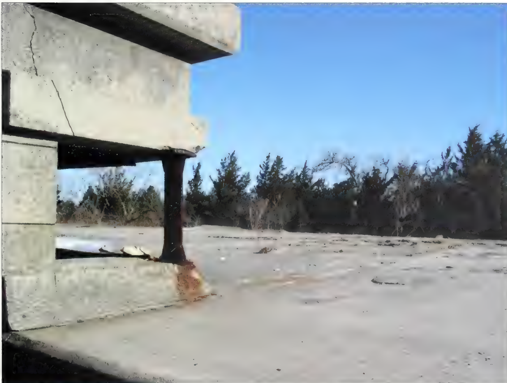
Figure 5.68. Blocked view northeastward from the battery commander's station at Battery Granger. Blocked downrange views to the water makes it difficult for park visitors to understand the historic operation of these coastal defense sites. Note corrosion of ferrous metal building features (Olmsted Center, January 2009).
